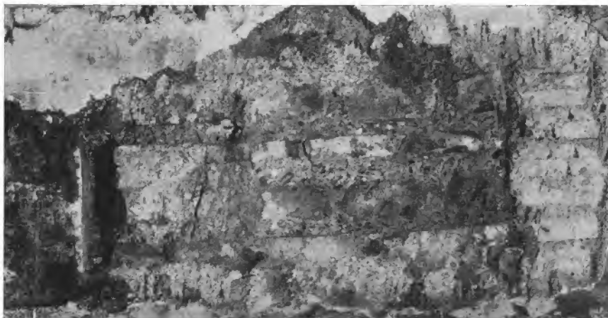
Fig. 156 — S. Lorenzo in Lucina. North wall of room to west of chancel. Right, fragment of brick wall. Center, opus listatum (Photo: Sansaini).
